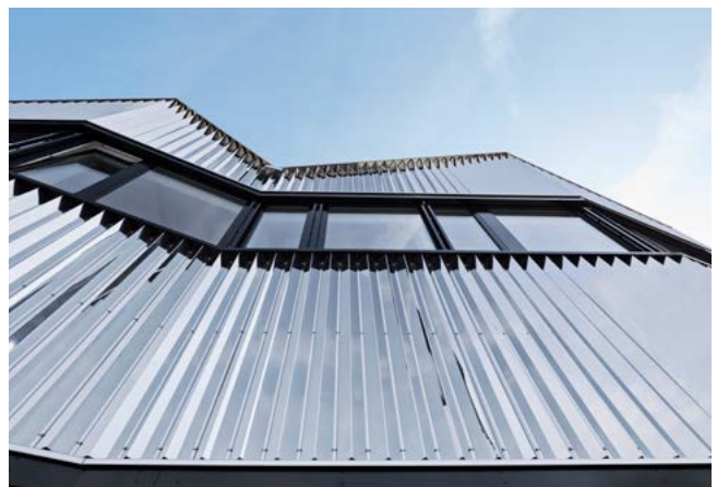
Building facade with Sandwich panels, using SFS SXC drill fasteners in the fastening process.
